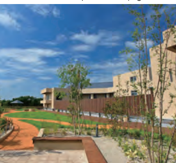
Hospital rooftop garden
